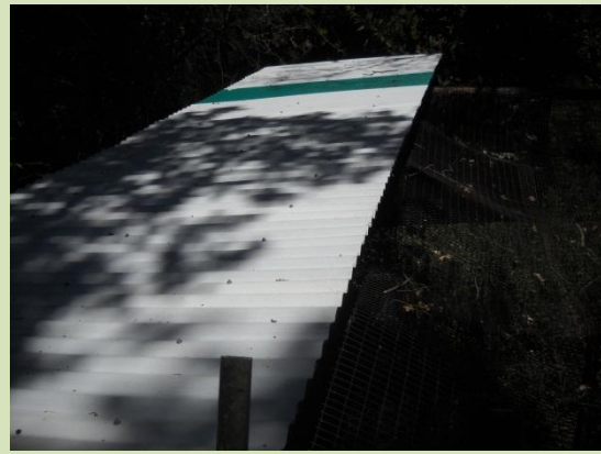
New Roof for The Flight Cage
