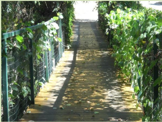
New Foot Bridge Wood Covering
