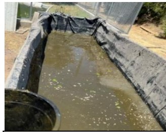
Dirty, sludge filled biofilter
